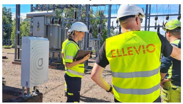
Currently, the project has been focused to the measurement and monitoring of  $SF_6$  gas at one of Ellevio's substations in central Sweden. However, by connecting more sensors to the SIPP Hub, the solution can be used in virtually all areas. The data gathered will provide network owners with an immediate insight into the need for maintenance, while also detailing other factors that could impact on operational reliability.
